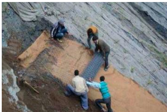
(Pictorial plan of the walls, grid beams, jute matting & GI mess laying)
