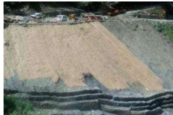
(Pictorial plan of the walls, grid beams, jute matting & GI mess laying)
